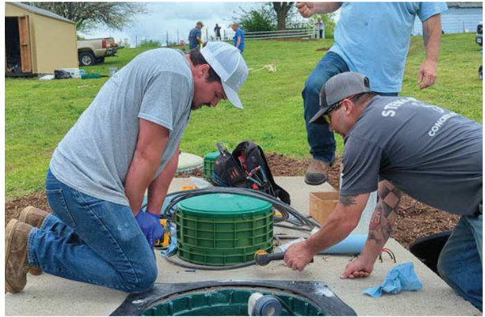
Jay helping replace aging risers at the Onsite Wastewater Training Center in Springfield.
