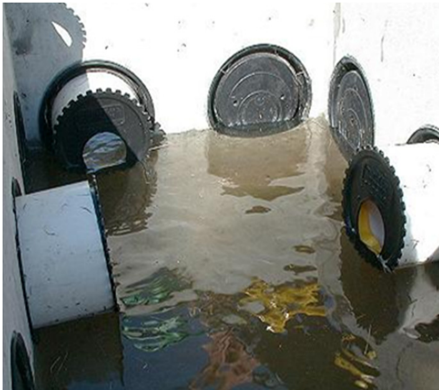
Using adjustable rings to adjust flow into D-Box.
