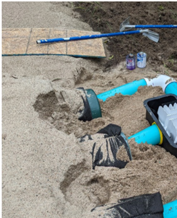
D-Box installation on AES System.
